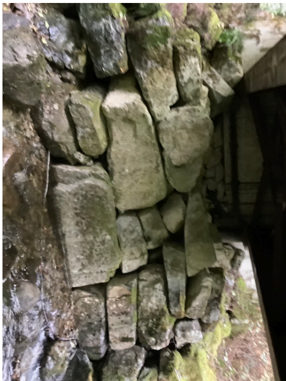
Left Bank Abutment when facing downstream
